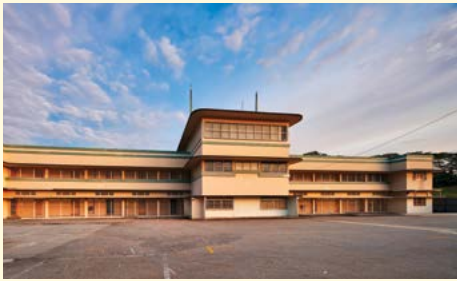
4 Former KD Malaya Administration Block
