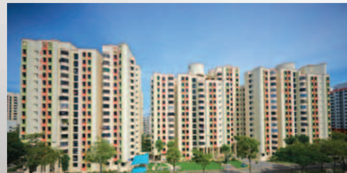
Newly repainted blocks in Canberra division: Blocks 339A-B, 340A-B, 341, 341A-B, 356A-C, 357, 357A-C, 359, 359A-C, 360A-C, 467, 467A-B, 468A-D, 469, 469A-B
