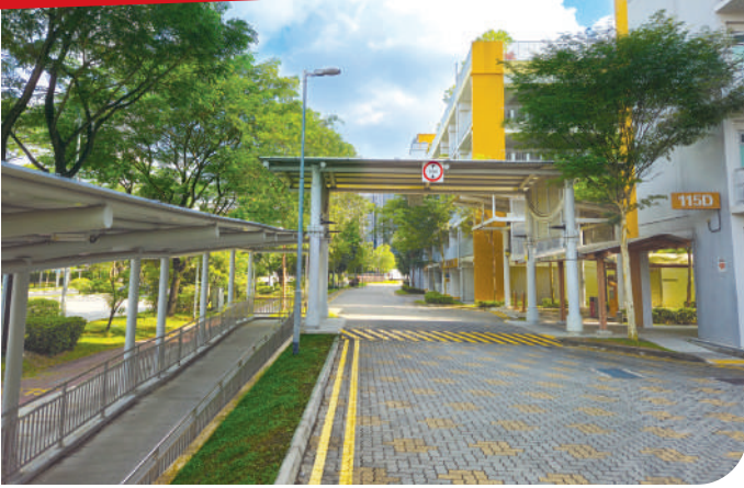
Upgraded Linkway at Blk 115D Canberra Walk
