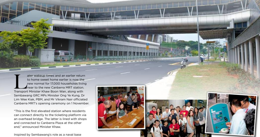
Inspired by Sembawang's role as a naval base in the past, Canberra MRT station's exterior is designed like a ship. Gentle wave-like forms along the roof welcome incoming trains, while curved metal louvres not only mirror the appearance of a ship's hull, but also facilitate ventilation. Glass panels that line the sides of the station let natural light into the station. An art installation titled Symbiosis, by artist Ms Tan Zi Xi, features aquatic flora and fauna as well.
