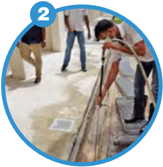
Drain flushing
