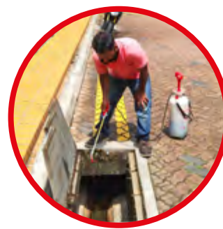
Oiling of drains
