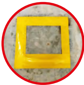
Sealing lightning protection system covers
