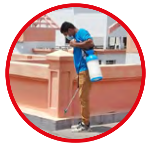
Inspecting rooftops to remove and treat all potential breeding grounds with insecticide
