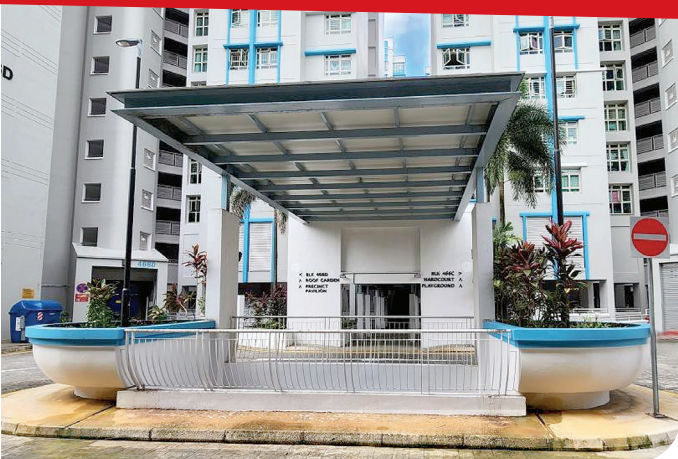
Upgraded Existing Drop-off Point from Blk 466C to 466D Sembawang Drive
