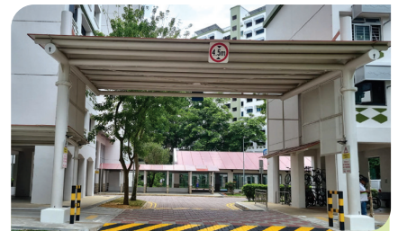
Naval Base Construction of High and Low Covered Linkway from Blk 402 to 405 Admiralty Link
