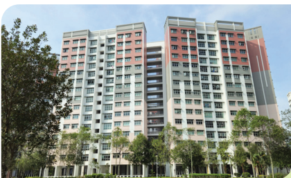
Sembawang Central Repair and Redecoration at East Brook @ Canberra
